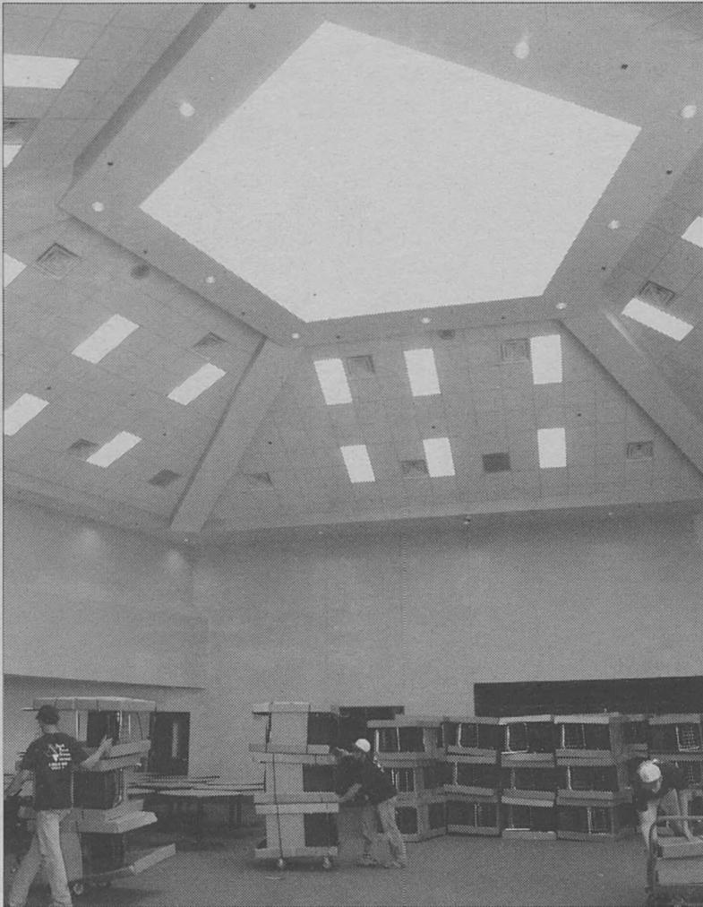
The completed cafeteria with workers getting the furniture ready.
